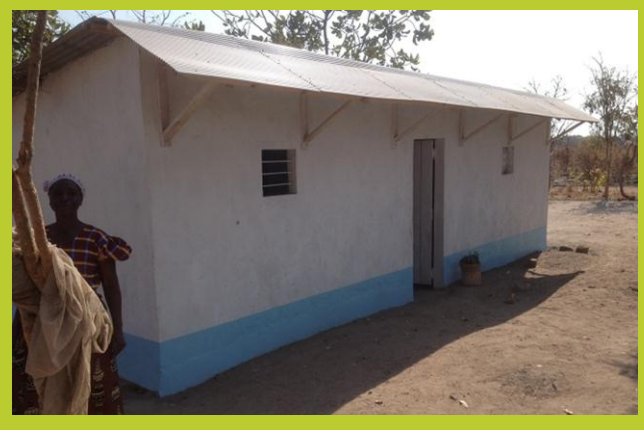
External walls of the birthing clinic and school will be rendered with cement to protect the mud brick work from the wet season rainfall.
