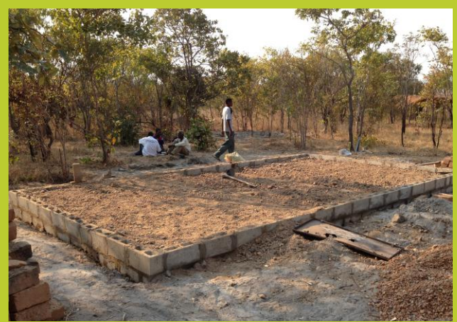
A local kiln is used to bake the bricks. Women used their hands to dig out gravel, taking 4 hours to gather a trailer load. TTN team members and community members dug trenches to begin foundations for the new clinic and school buildings.
