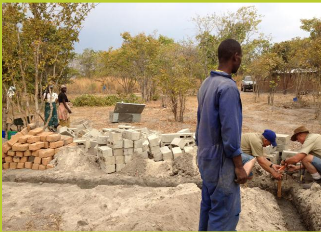
A local kiln is used to bake the bricks. Women used their hands to dig out gravel, taking 4 hours to gather a trailer load. TTN team members and community members dug trenches to begin foundations for the new clinic and school buildings.
